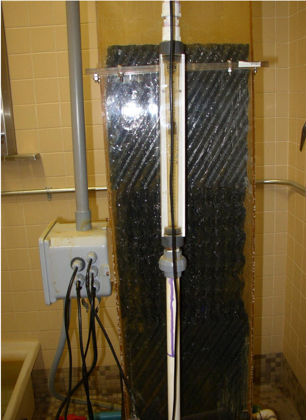
Figure D21 – T1 (Control) prior to PEFD Trial 1/2. Packing has been replaced and seasoned
