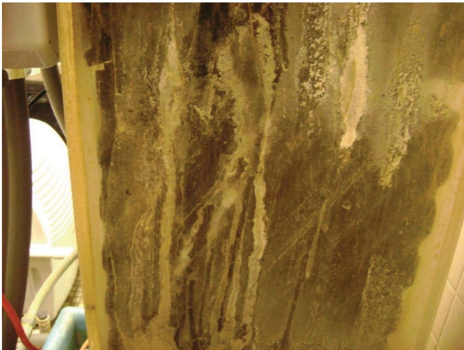
Figure H32 – Close-up of T2 (Device) following HCD trial
