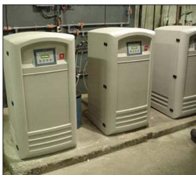
Multiple chlorine dioxide generators can be installed to accommodate larger demand or to provide backup units.
